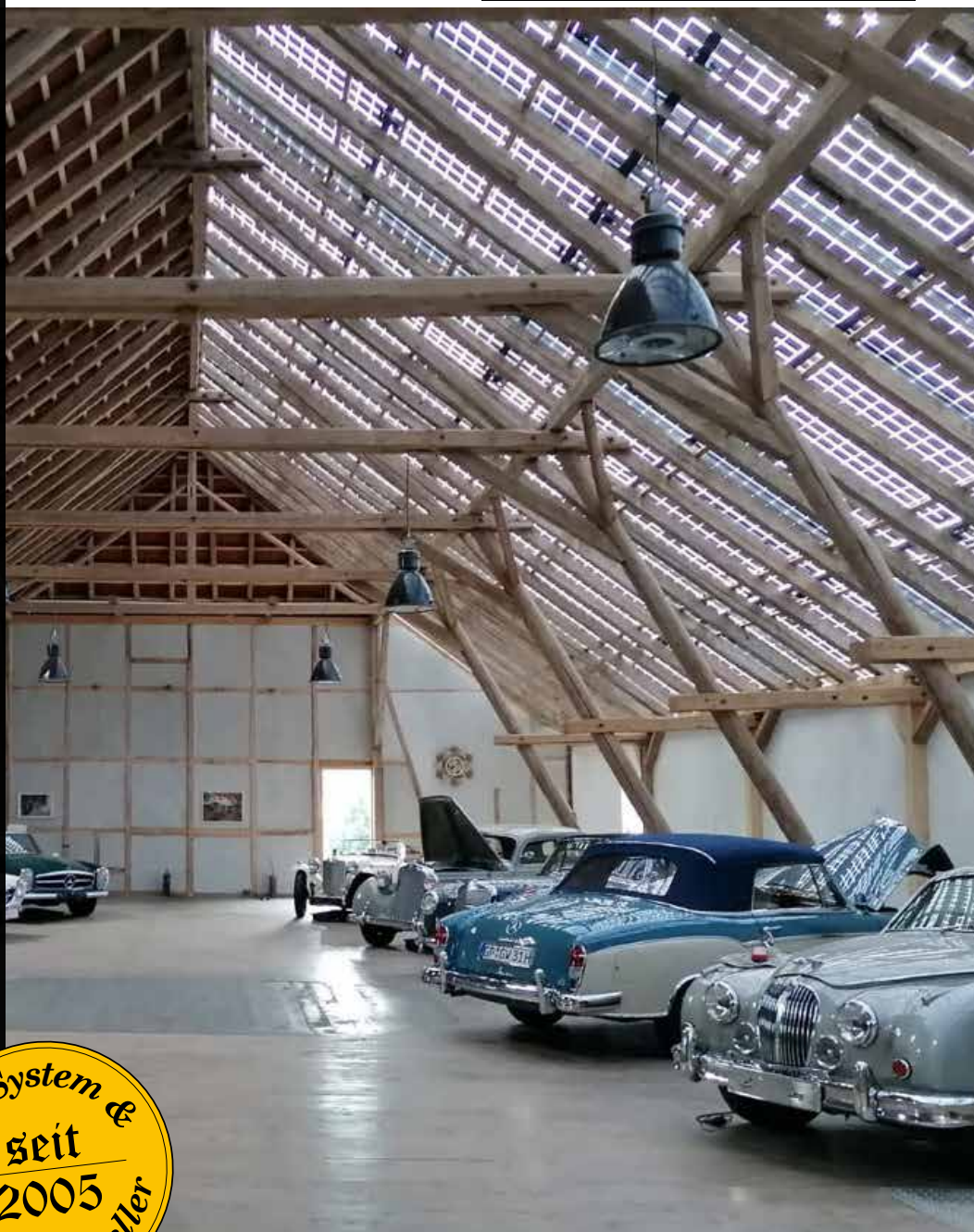
2022 / Scheune GS-Module / 48,40 kWp
